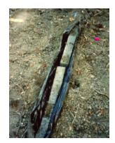
**Figure 7** Root barriers made of unit pavers wrapped in plastic.
