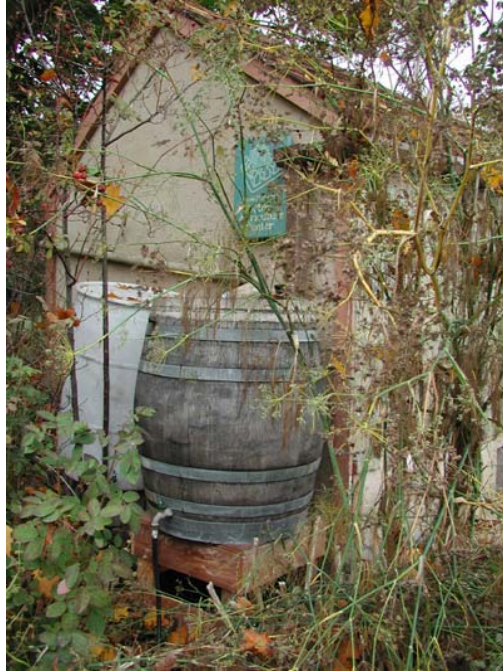
Rain barrels collecting water from tool shed roof
