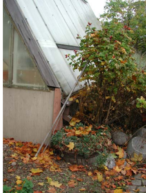
Stormwater planter collecting water from greenhouse
